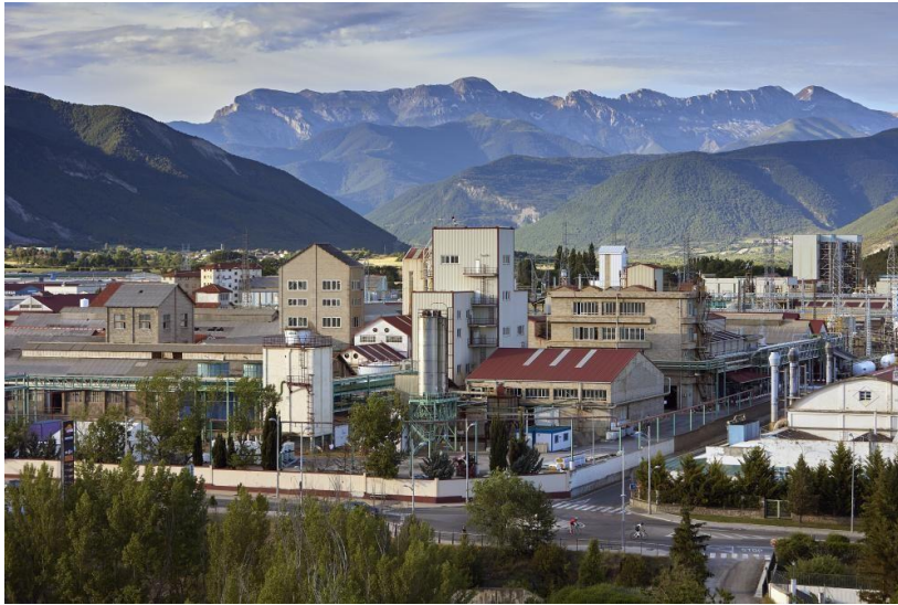
General image of the Sabiñánigo factory
