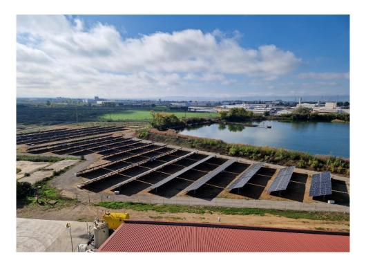
The new photovoltaic plant installed at the Ercros factory in Monzón (Huesca) reduces  $CO_2$  emissions by 220 tonnes per year. Its power is 750 kWp and its generation capacity is 850 MWh/year.
